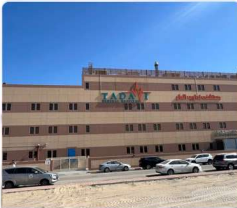
04 TADAWI HOSPITAL Dammam, Saudi Arabia
